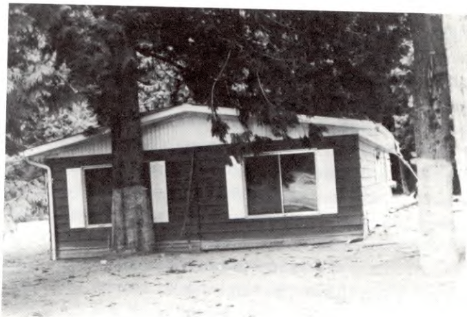
Figure 280.—Locally passive nature of mudflow is shown by relatively intact condition of house, which apparently floated on mudflow surface to this position.
